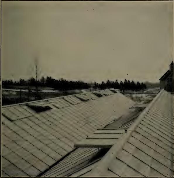
12—Roofs of twelve foot houses, showing method of construction and of attaching ventilators; one row of glass between the ventilators.
